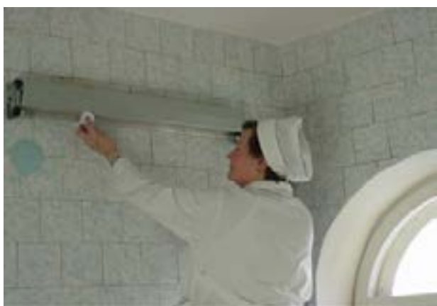
Fig. 3.6. Cleaning a GUV fixture in a health care facility
